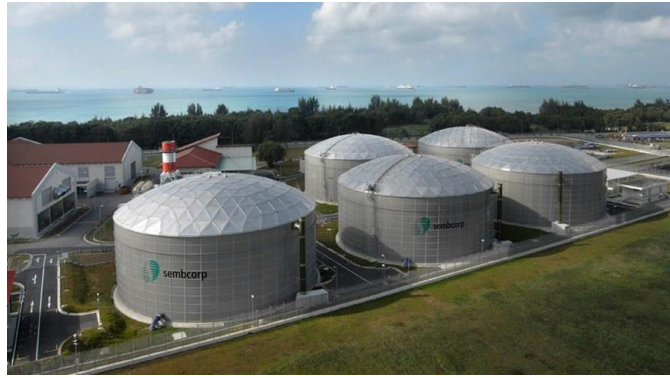
Figure 1: Sembcorp NEWater Plant in Singapore (Changi Water Reclamation Plant & Sembcorp NEWater Plant, 2023)
