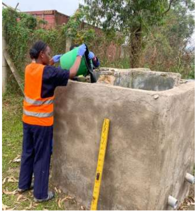
Figure 26: Pouring sludge in the sludge bed
