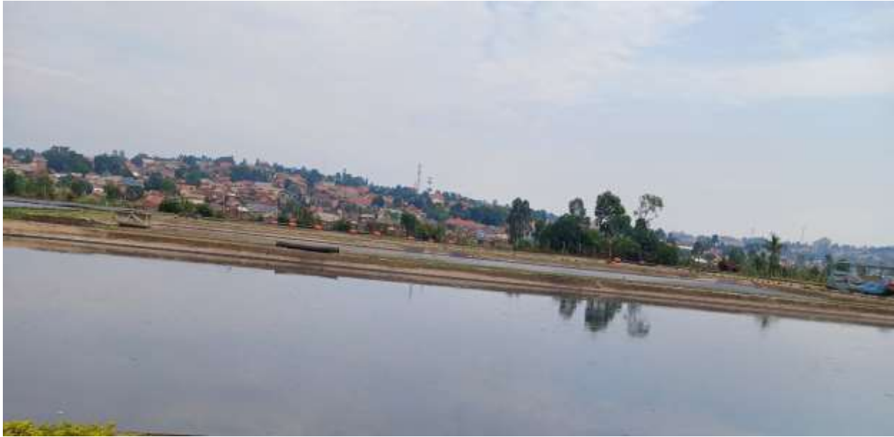
Figure 10: Anaerobic ponds at secondary stage of treatment.
