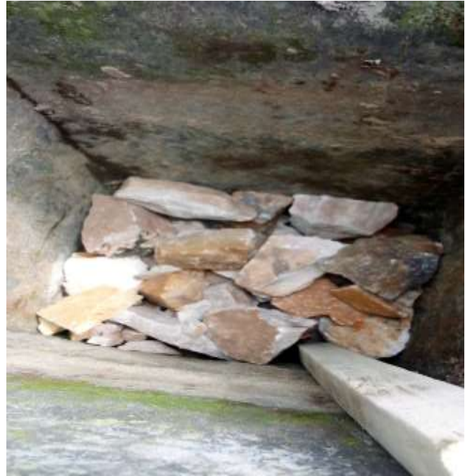
Figure 22: Layer of hardcore in filter media
