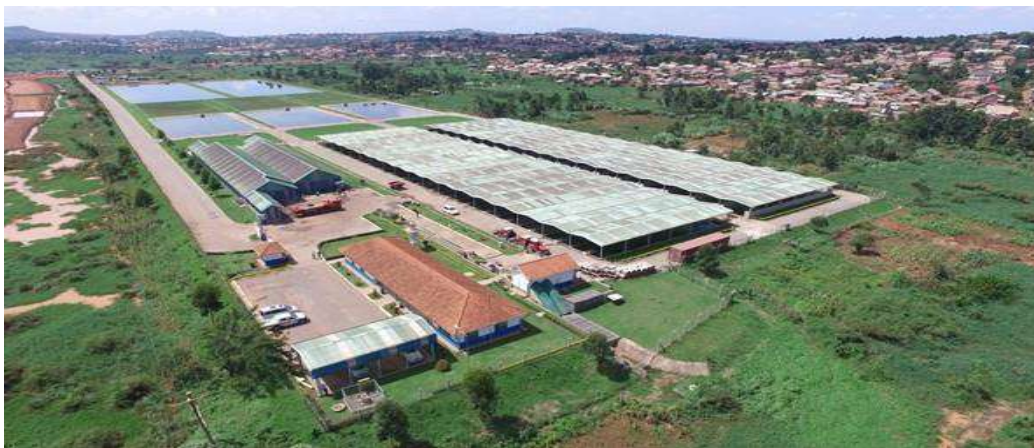
Figure 1: An Aerial View of Lubigi Treatment Plant. (NOBLE, 2021)
