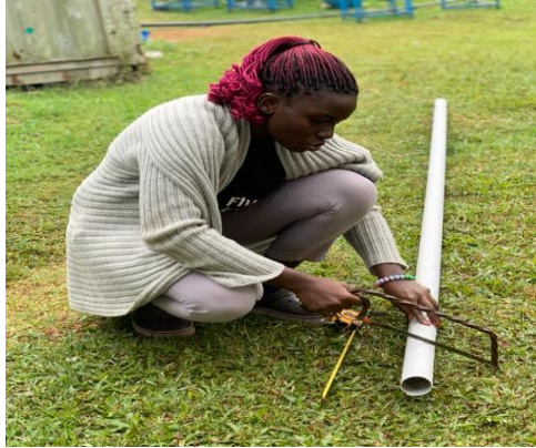
Figure 11: cutting of Pipe for Digester inlet
