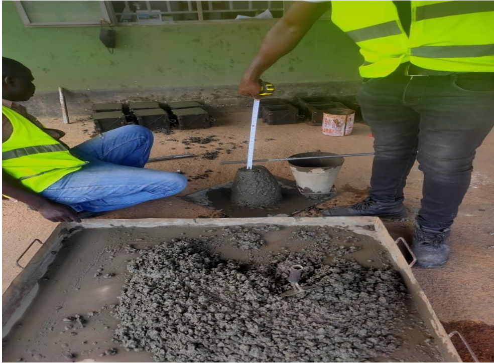
Figure 4: showing slam test of 5% SCBA Concrete mix
