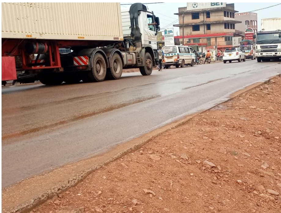
Figure 1: Climbing lane section on Kampala - Jinja road.
