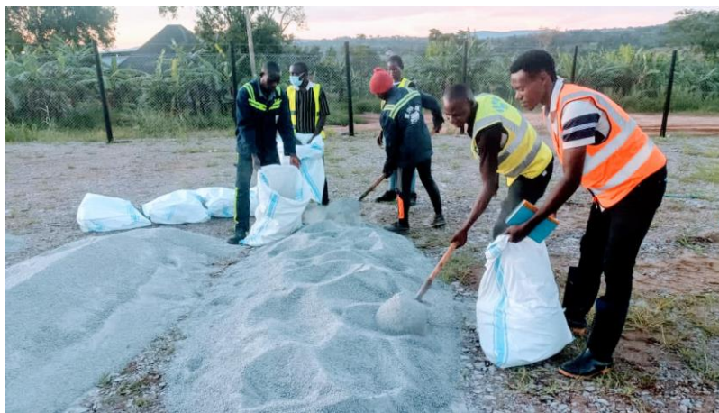
Figure 12: Acquiring aggregates from Wankoba quarry site
