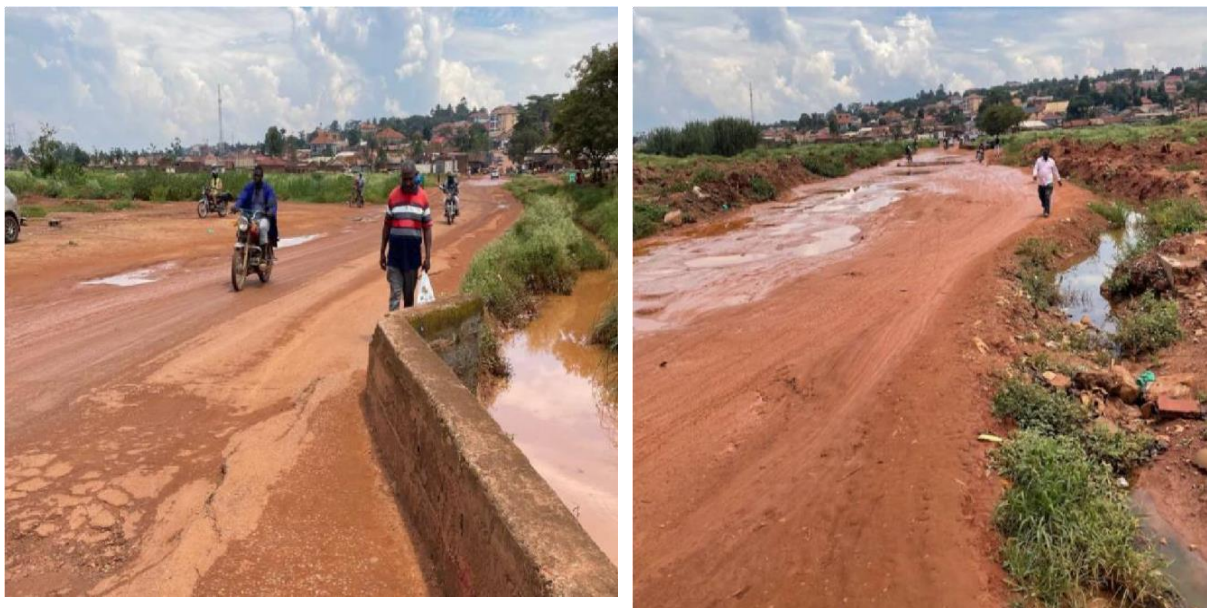
Figure 1. 1 Current condition of the roadside drainage
