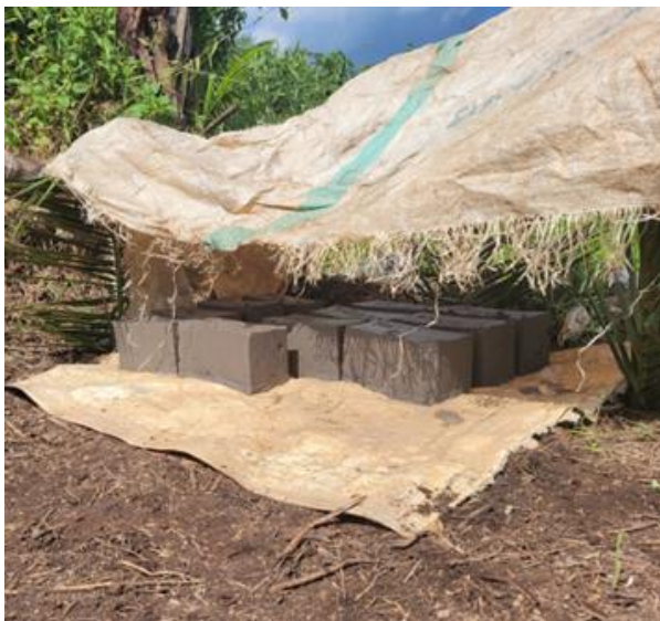
Figure 22 Curing of the stabilized bricks
