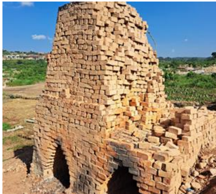
Figure 1: A Fire-burnt brick production kiln at Ntawo brick laying site
