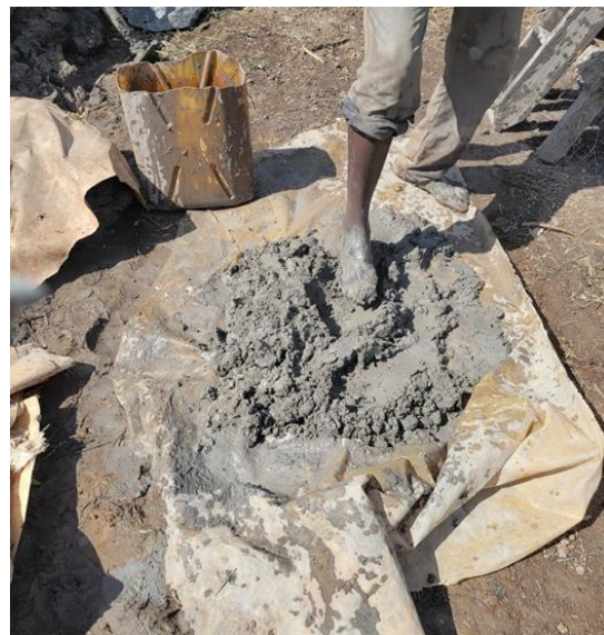
Figure 23 Mixing of the RHA into the soil
