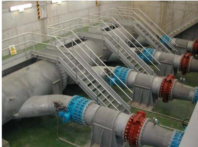
Figure 10: A Reclaimed water pumping station for instream flow and agricultural irrigation (Mujeriego et al., 2008).
