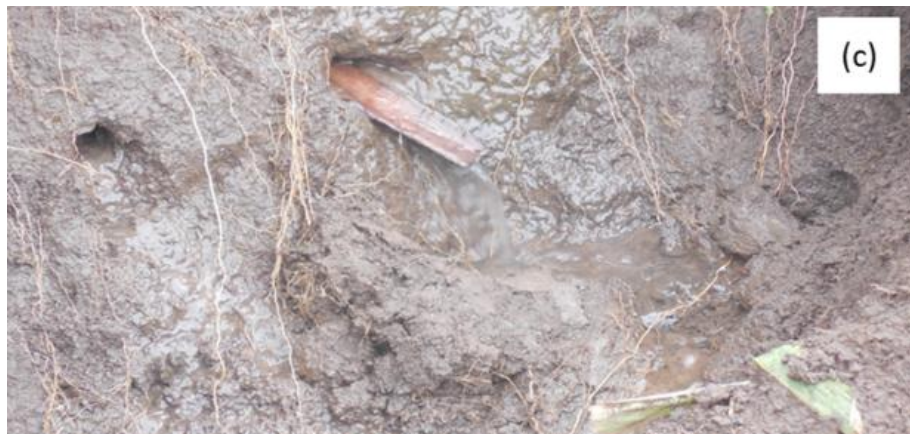
Figure 7. Natural dewatering of the gully the bank with installed sub-drains.
