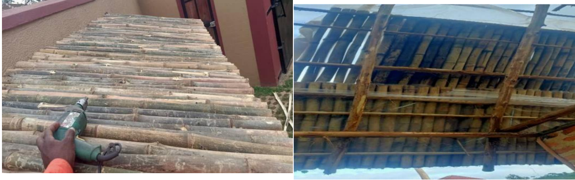
Figure 1: Bamboo roof structure
