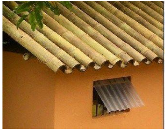
Figure 12: Showing a bamboo roof sample after treating with epoxy resin
