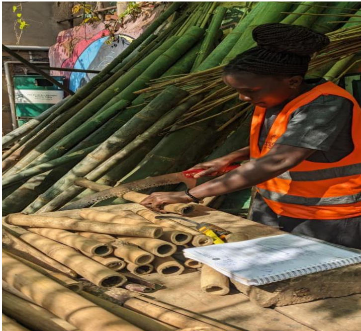
Figure 3: Preparation of Bamboo through culm cutting
