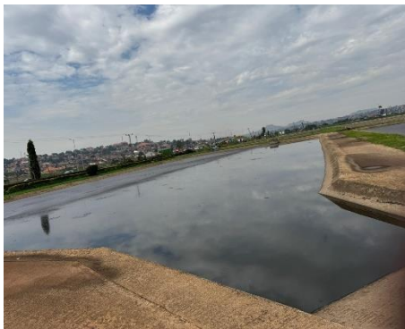
Figure 5 Aerobic pond
