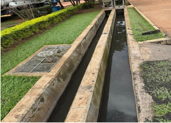
Figure 3 Grit chamber
