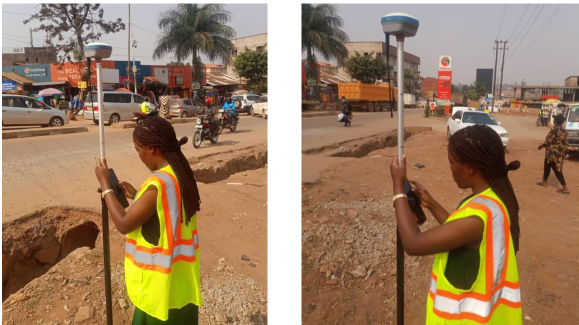
Figure 18: Collection of topographic data
