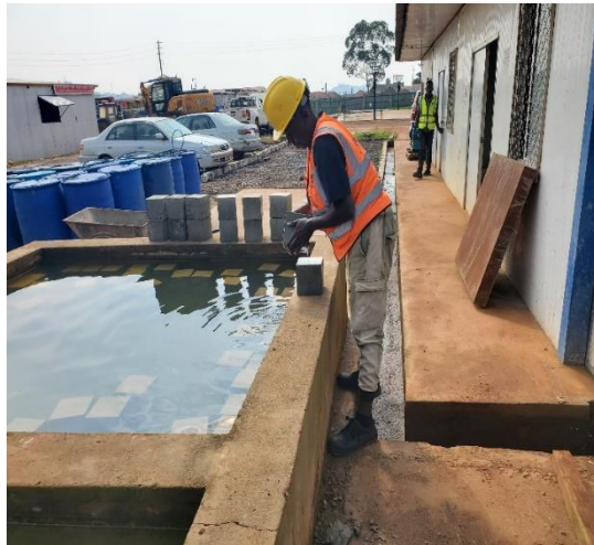
Curing of cubes
