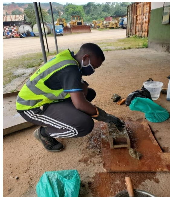
Figure 10: Molding of the final brick product
