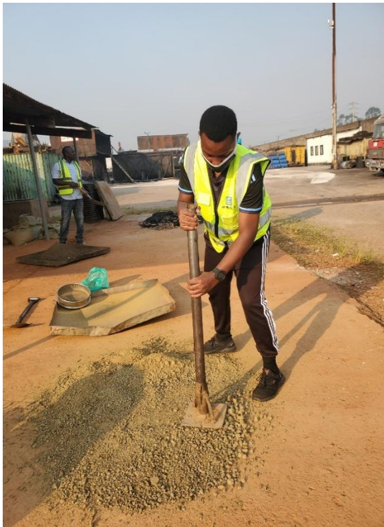
Figure 9: Pre-crushing of the semi-dry clay material in preparation for brick making
