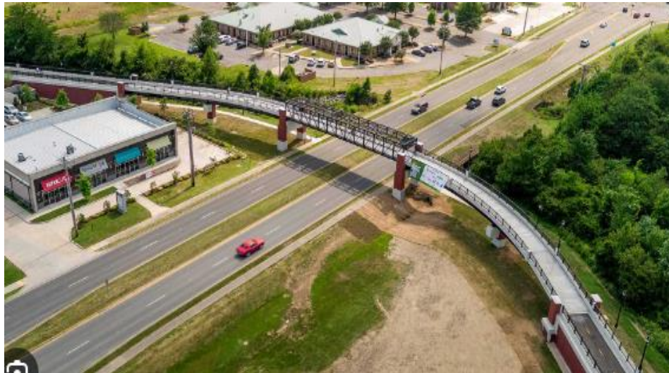
Figure 4: An Overpass (Source: Dave Creek)
