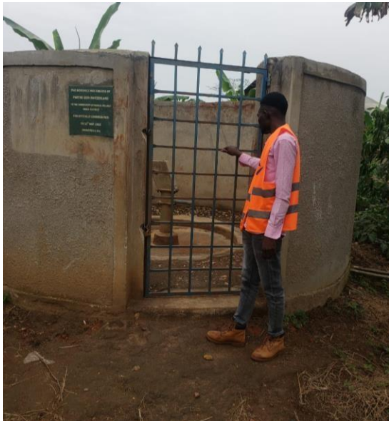
Abandoned borehole due to high iron
