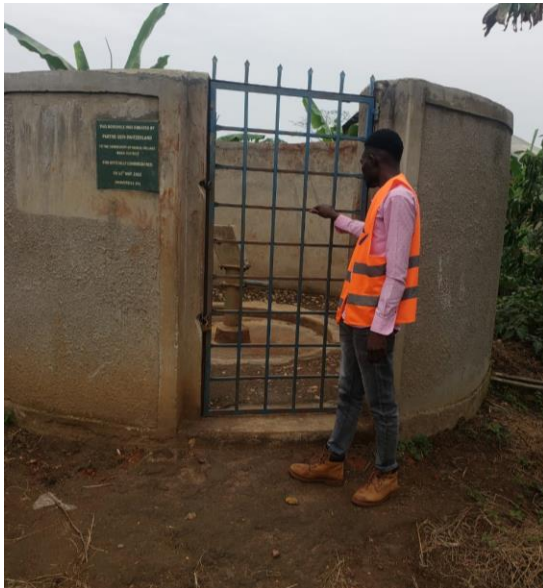
Abandoned borehole due to high iron
