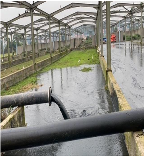
Figure 20: Freshly pumped sludge
