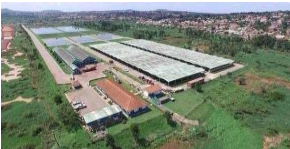
Figure 1 : An Aerial View of Lubigi Treatment Plant (Wasswa, 2022).
