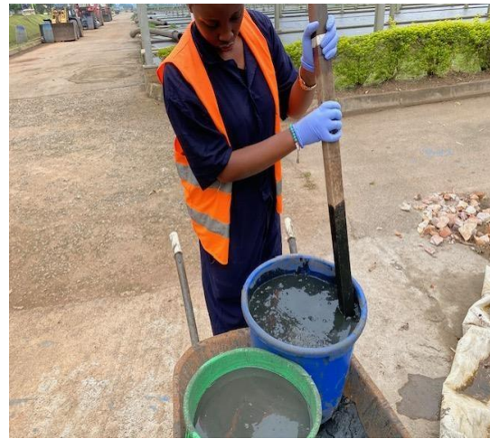
Figure 10: Mixing FS with rice husk ash
