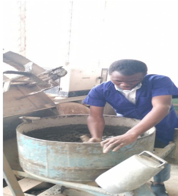
Appendix Figure K-6: Mixing of concrete manually
