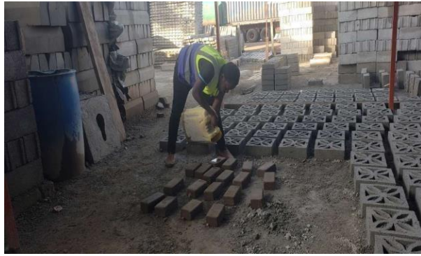
Figure 24: FRESHLY MADE CONCRETE PAVERS WITH POLYESTER FIBER BLEND AS REINFORCEMENT
