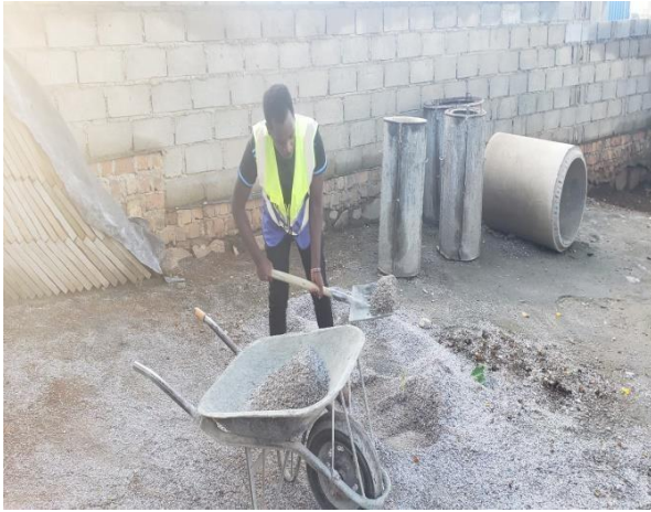
Figure 6 showing coarse aggregate being collected for mixing
