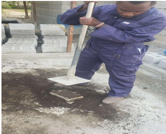
Figure 22: FOUNDRY SAND SIEVED AND READY FOR CASTING OF THE CONCRETE MIX
