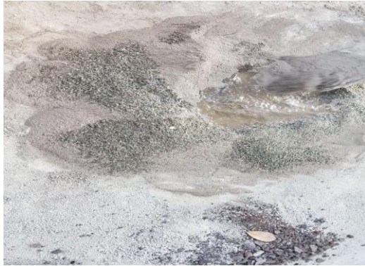
Figure 20 Figure 21 CONCRETE MIXING WITH APPLIED FRACTION OF POLYESTER FIBER AS REINFORCEMENT.
