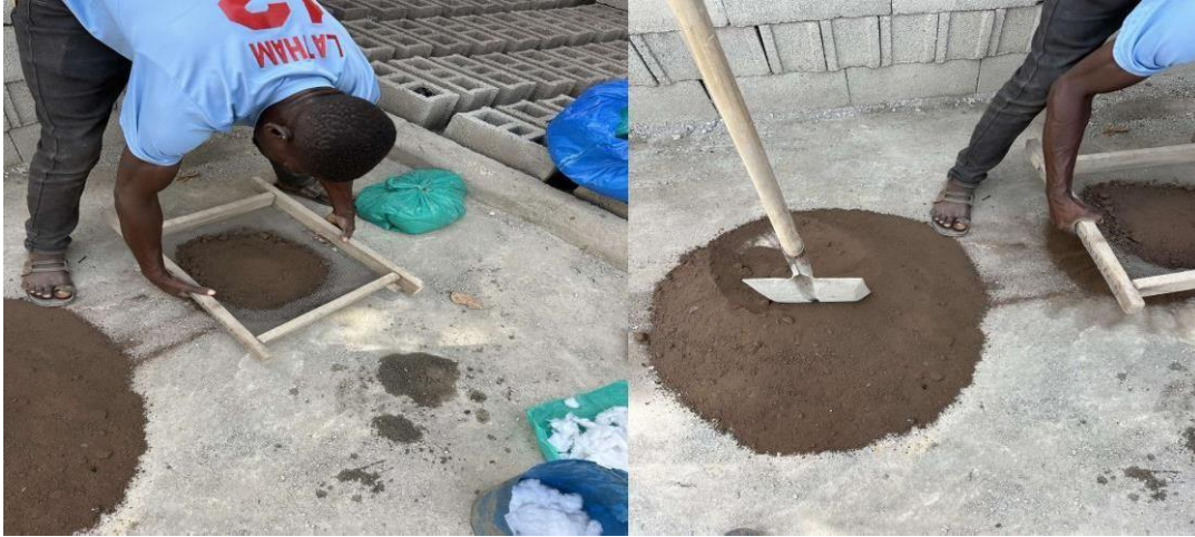
Figure 9: MIXING OF COARSE AGGREGATES INTO THE CONCRETE MIX
