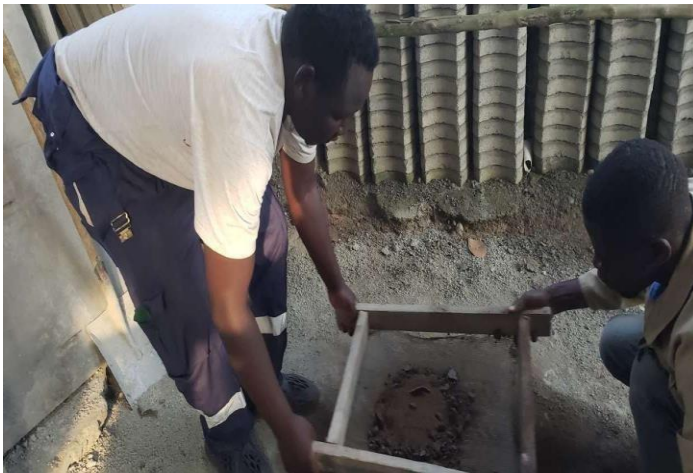
Figure 18: WEIGHING OF A REPRESENTATIVE FRACTION OF THE POLYESTER FIBER FOR OPTIMIZATION OF THE CONCRETE MIX
