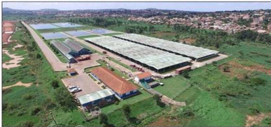
Figure 1: Aerial view of Lubigi treatment plant
