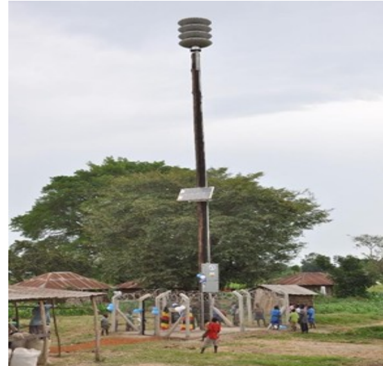
Figure 5.3: Solar powered siren adjacent to the river in Butaleja district.
